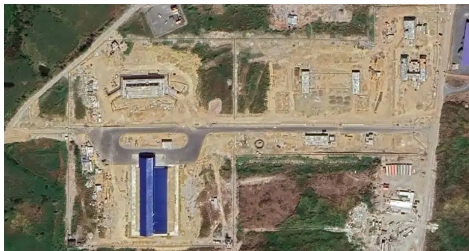
Construction of a BrahMos missile site at
