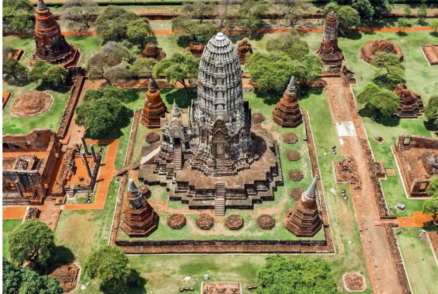
World Heritage Site of Ayutthaya , after its repair
