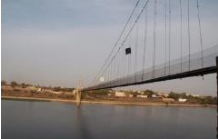
Morbi suspension footbridge
