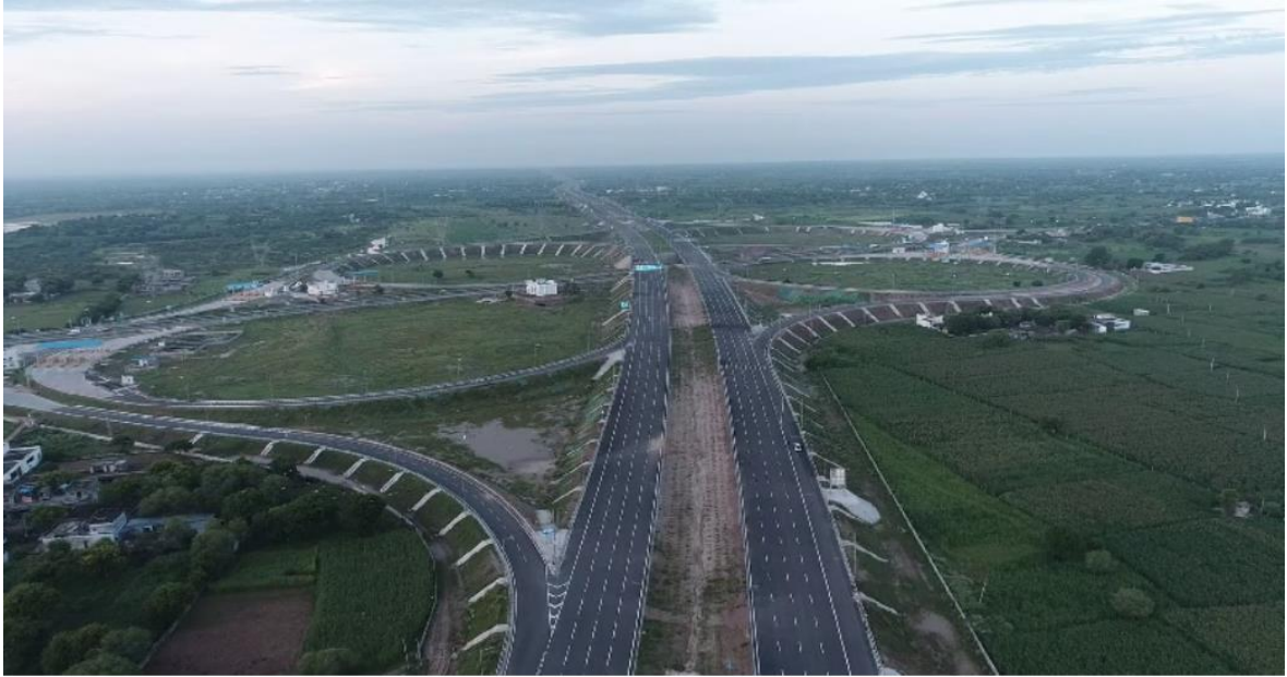
Delhi-Mumbai 4 lane Expressway
