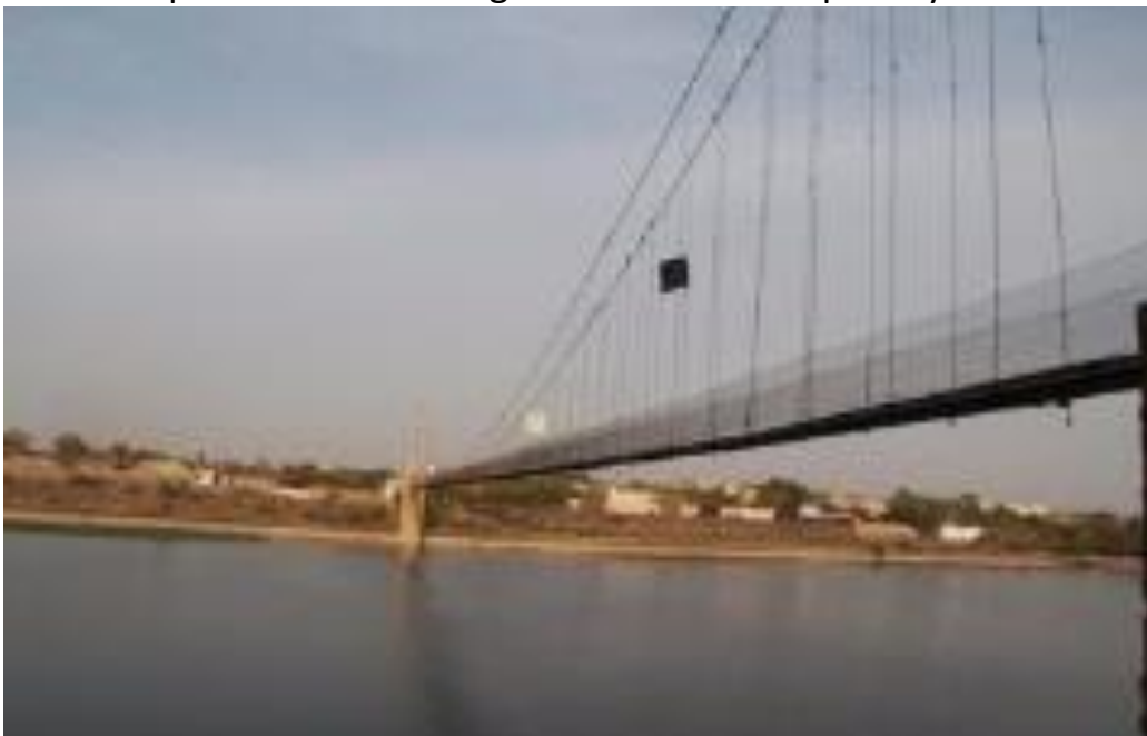
Morbi suspension footbridge
