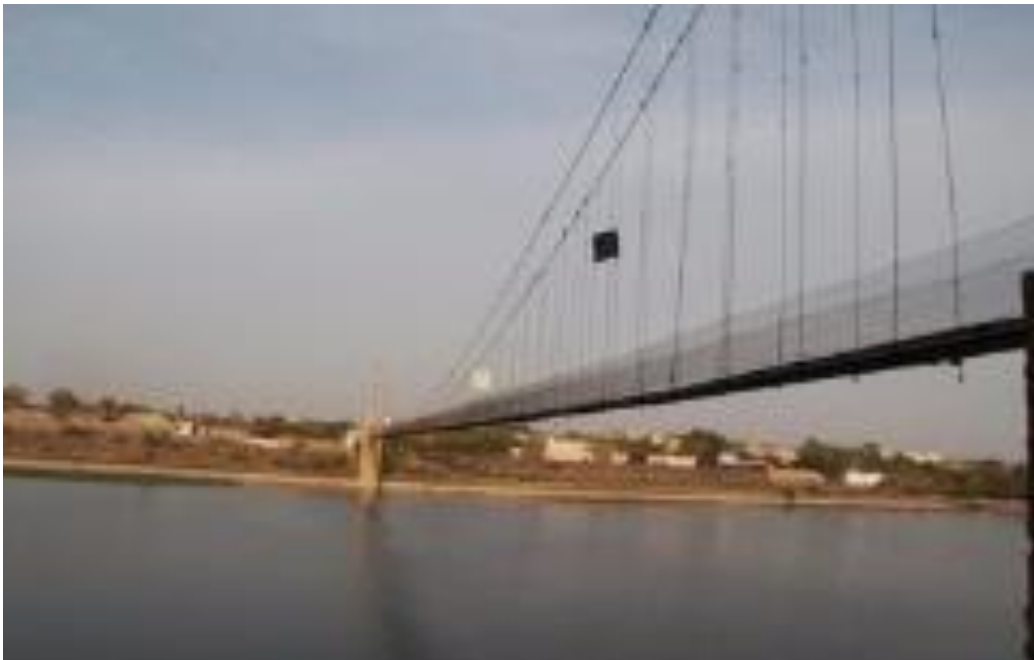
Morbi suspension footbridge
