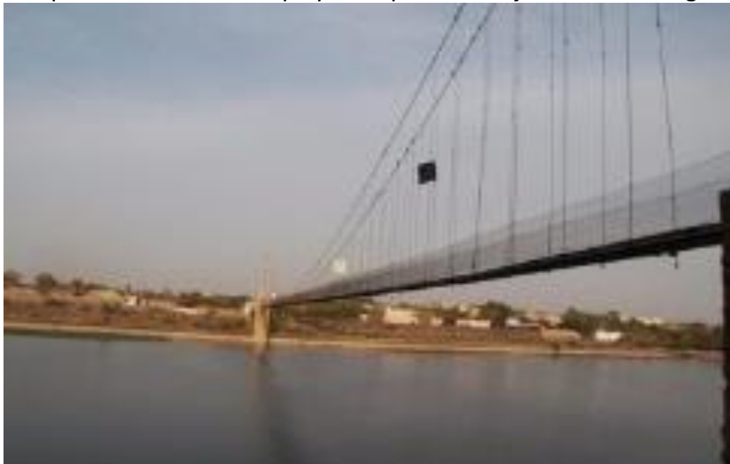
Morbi suspension footbridge
